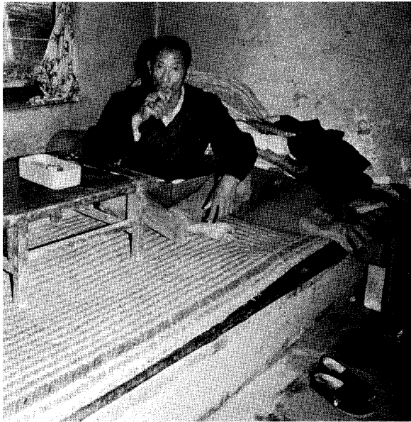
94 A Chinese kang brick sleeping platform with internal flues (near Beijing).
