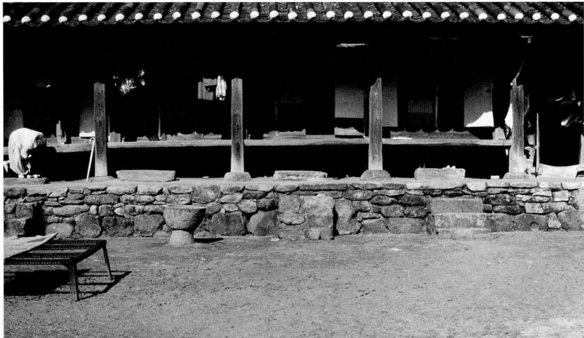
107 A view of the anmadang and the raised floor structure of the taech'ong .
