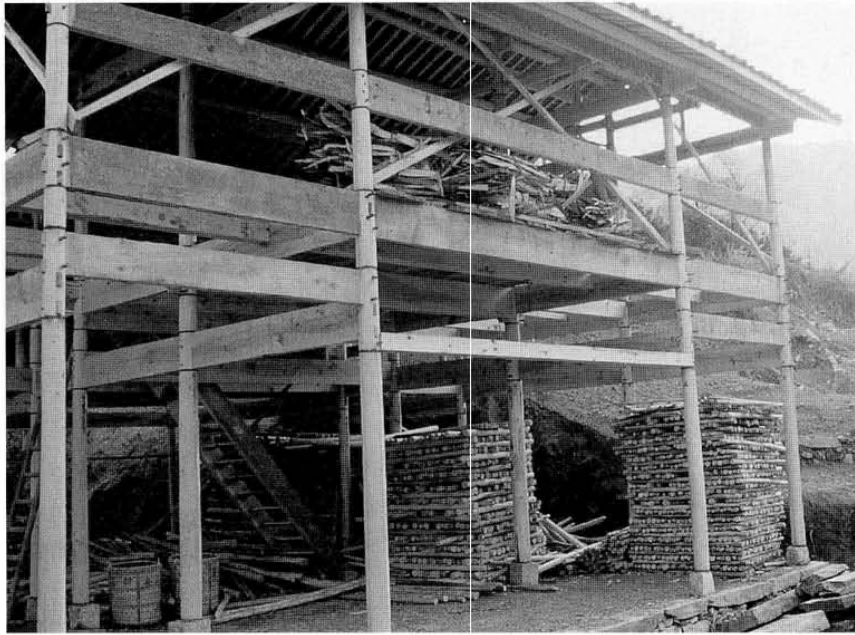
53.1 The wood-frame structure of a Huizhou dwelling.
