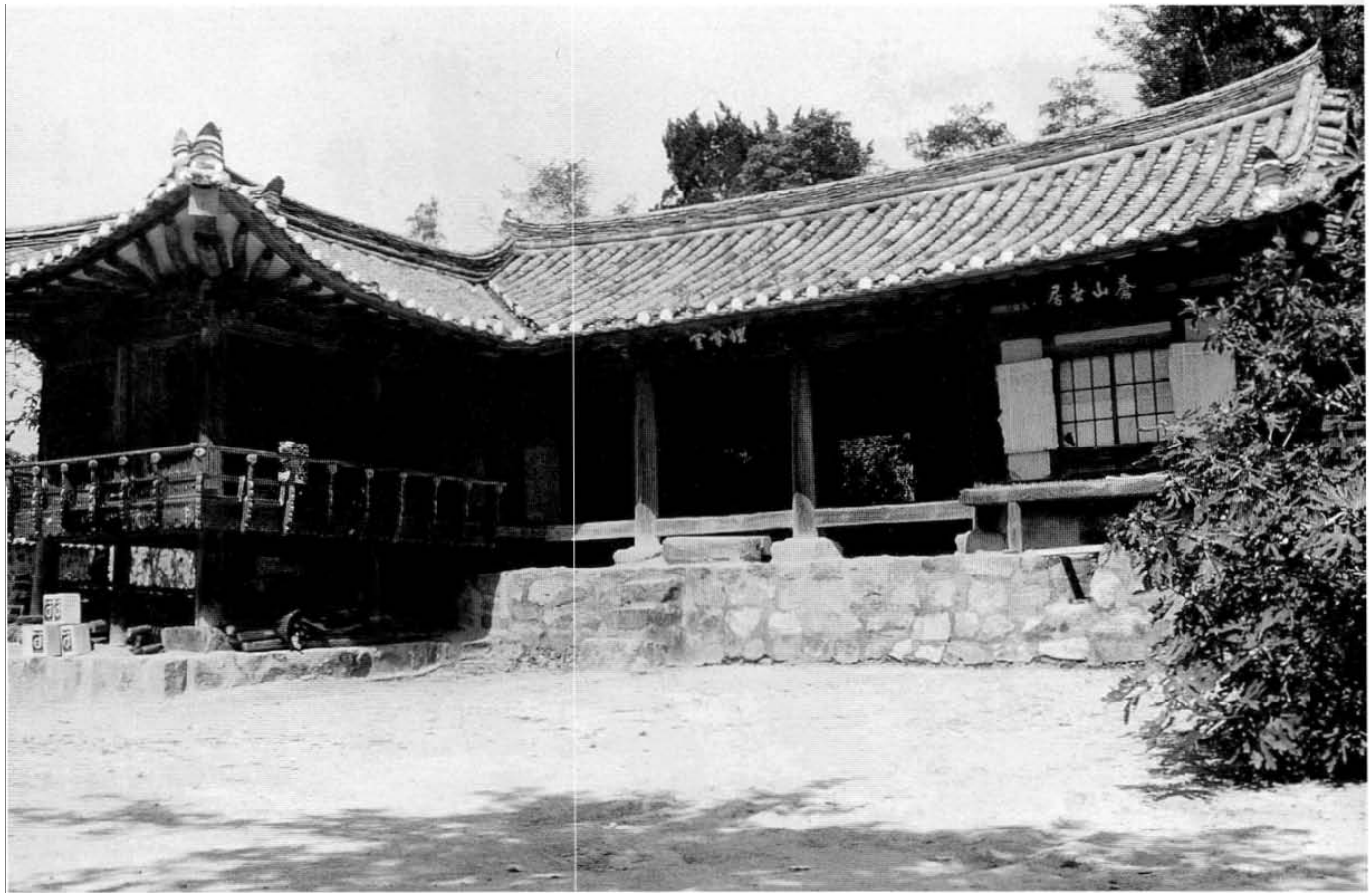
110.1 A sarangch'ae composed of (from left to right) a numaru , sarang taech'ong , and sarangbang (Mugongdang, Wölsöng).
