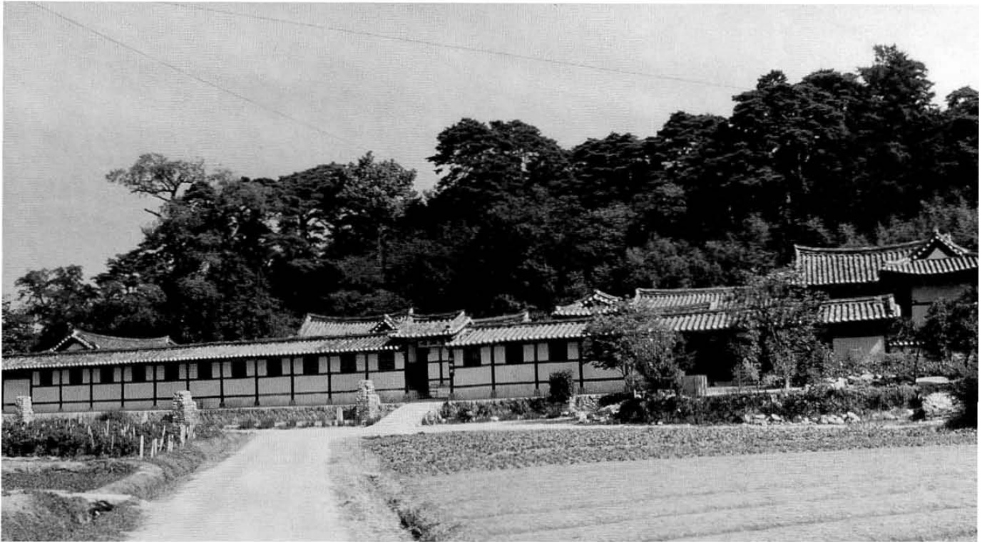
115.2 The Sŏn'gyojang exterior facade.
